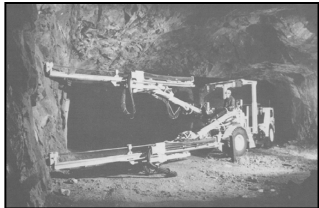
Mechanized Hydraulic Jumbo Drill
