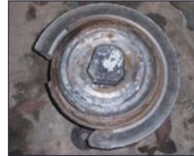
crack, brittle fracture
