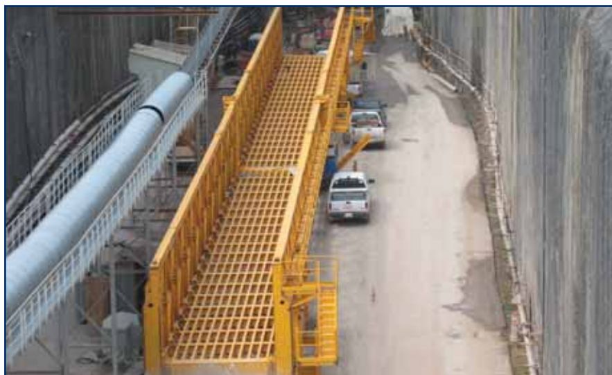
Figure 7: Invert Concreting Gantry Structure
