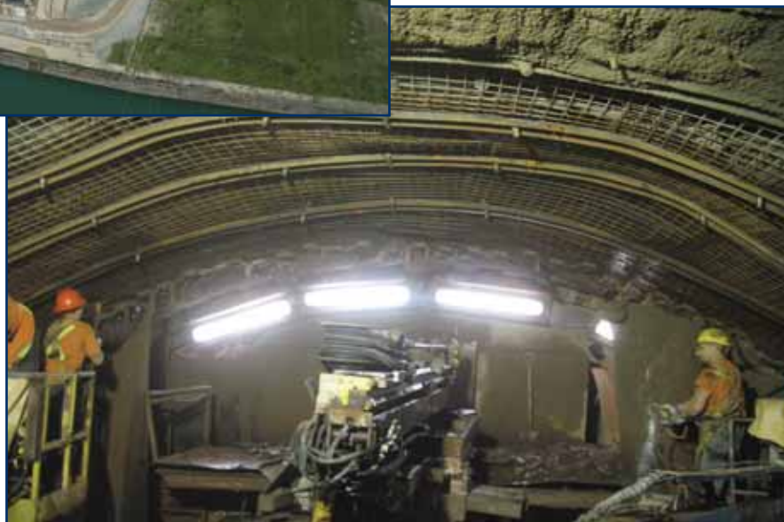
Figure 3: Rock Support Installation in the 'L1 Build Area'
