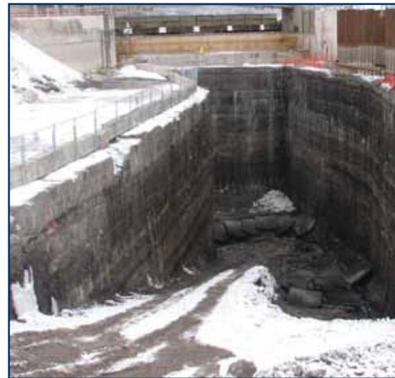
Figure 6: Intake Channel Excavation
