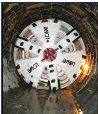
Typical TBM Head Dressing
