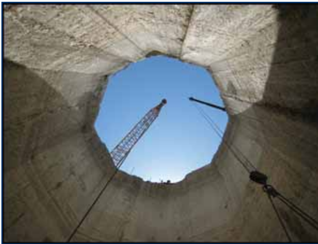
Slurry Wall Shaft – 19th Avenue
