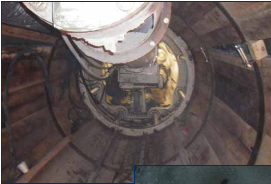
TBM jacking can and screw auger
