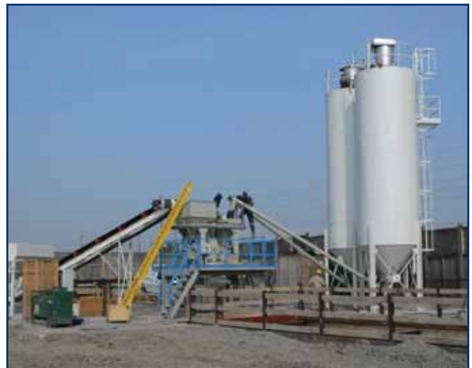
Tunnelling set-up – Langstaff
