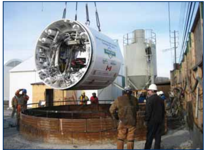
Installing first TBM Bathurst
