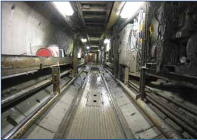
TBM and tunnel – 19th Avenue
