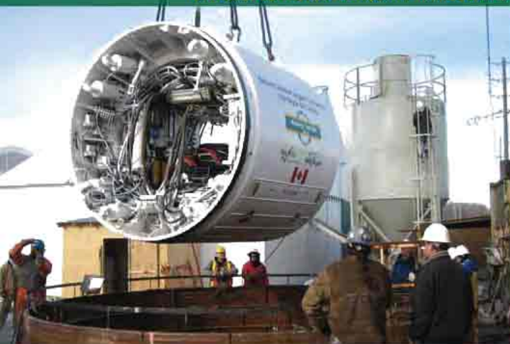
BATHURST COLLECTOR & LANGSTAFF TRUNK SEWERS
