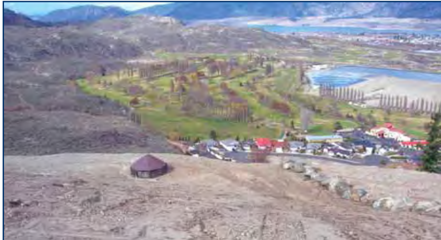
Final grading of the site.
