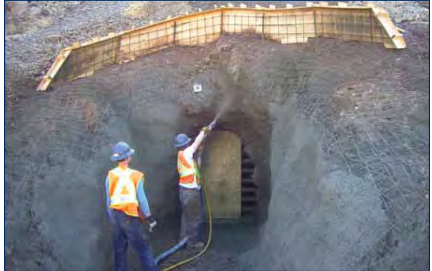
Portal two under construction.
