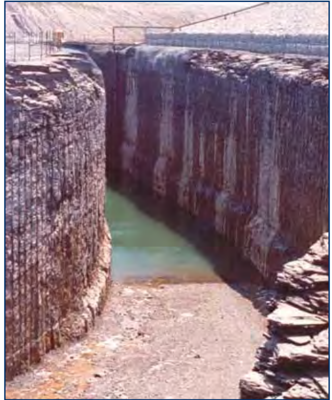
Figure 4. Forebay walls excavated by use of presplit blasting at Darlington
