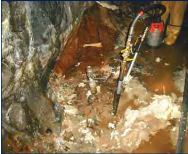
Grout plugs are installed to allow high pressure injection of Multiurethanes Universal Resin.
