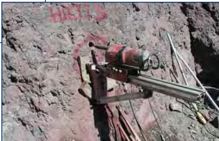
Figure 8. Hilti-drilling into outcrop
