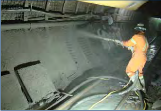
Figure 5. Final support as shotcreting
