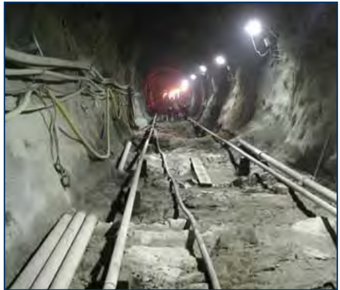
Figure 6 – Concrete Invert Works for D&B Tunnel
