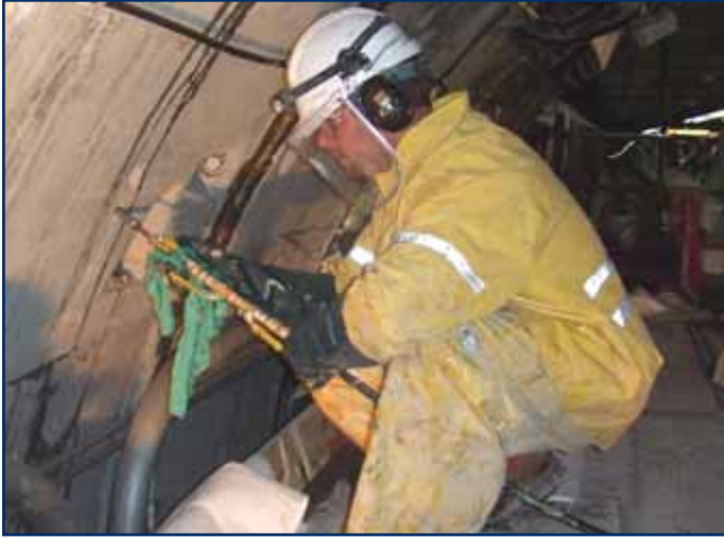
Technical grouting requires experience. Multiurethanes technicians can provide training for your team on grouting fundamentals.
