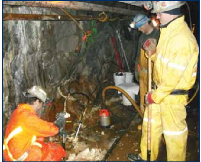
Flowing water makes tunnelling work very difficult. Multiurethanes has the experience and technical support to resolve challenging water cut-off situations.
