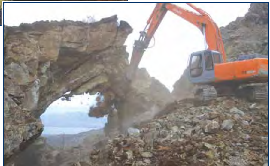
Rock breaker removing a pillar.
