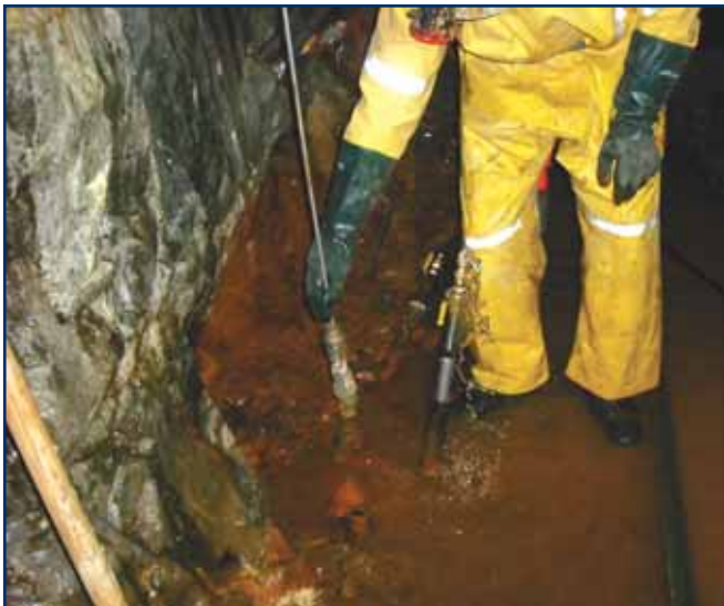
Experienced grouting technicians work together to stop the most difficult water flows.
