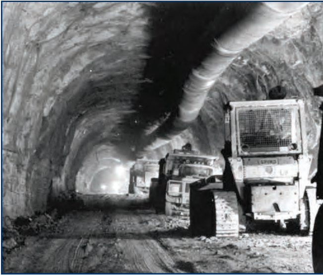
Figure 3. View of tunnel at Darlington
