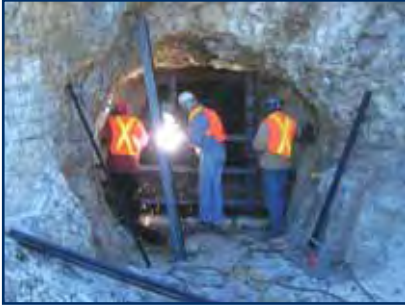
Constructing a bat gat at portal one.
