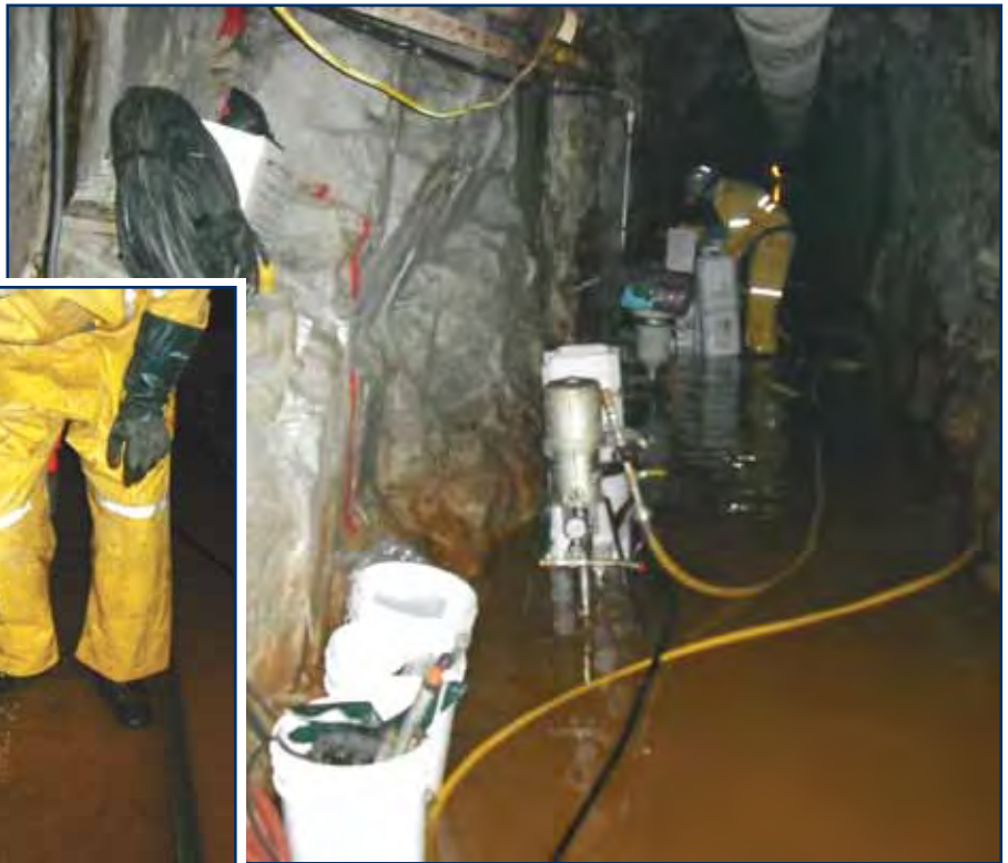
From high volume flowing water to a dry tunnel. Call Multiurethanes when difficult ground conditions are experienced on your jobsite.
