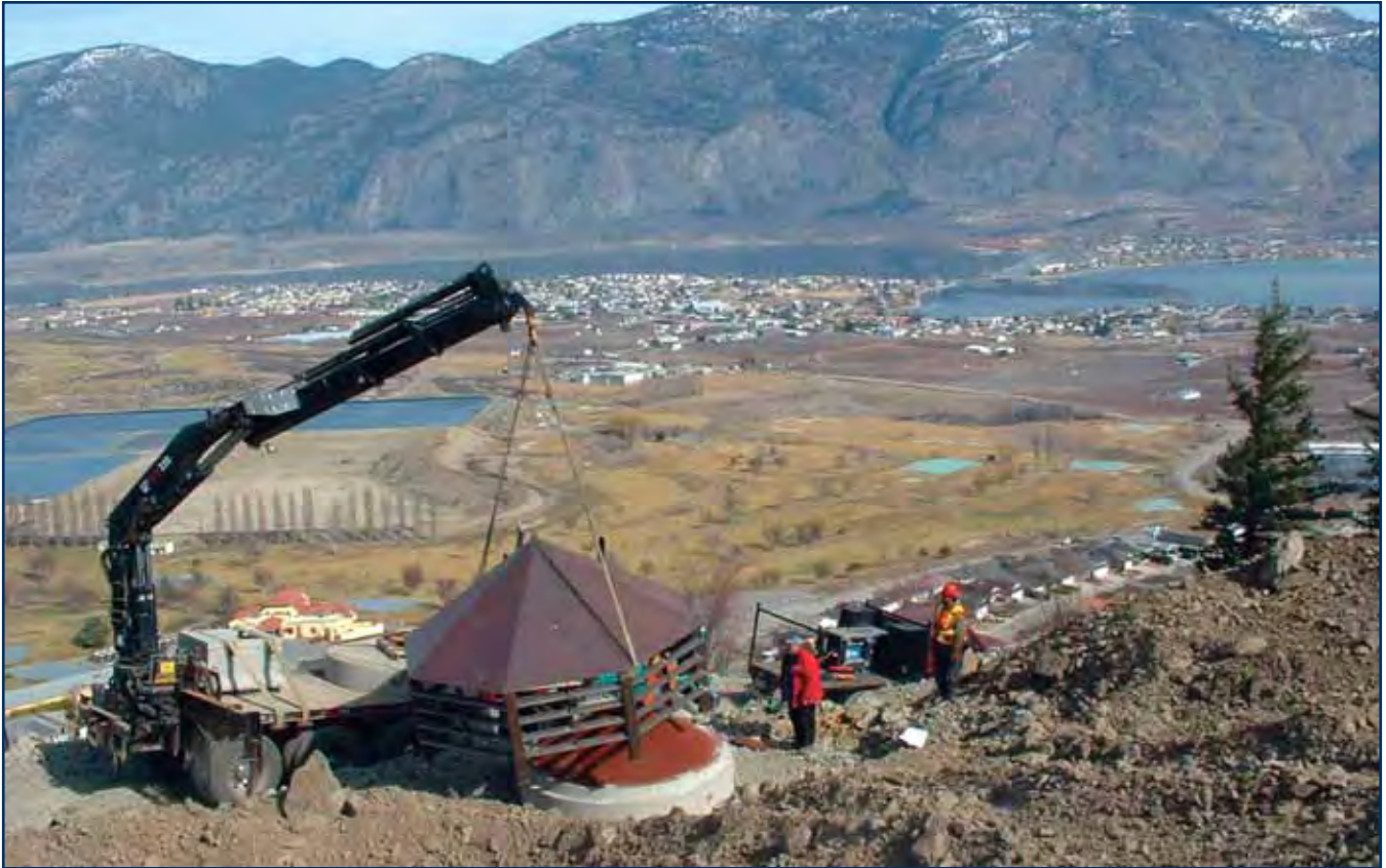
Bat vent installation.
