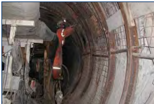
Figure 4. Support installation in small TBM tunnel
