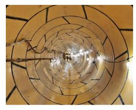
Combisegments® from Herrenknecht Formwork meet the need for future-proof and reliable concrete protection in tunnelling with the segmental lining process. Combisegments® are corrosion-resistant and hydraulically optimized segments that are fitted with a Combisegments® protective lining and an integrated sealing frame during production.
