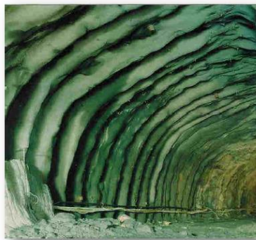
Left: Appearance of ('bent') RRS in subway station location where central pillar was excavated after side-cuts.
