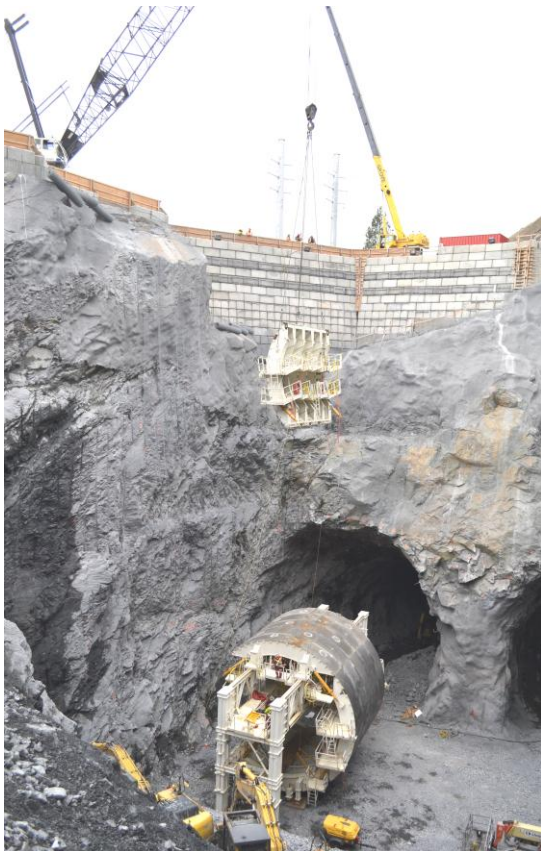
Figure 5. Tunnel form re-assembly in bottom of intake excavation.
