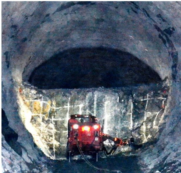
Figure 3. Top heading and bottom bench excavation.
