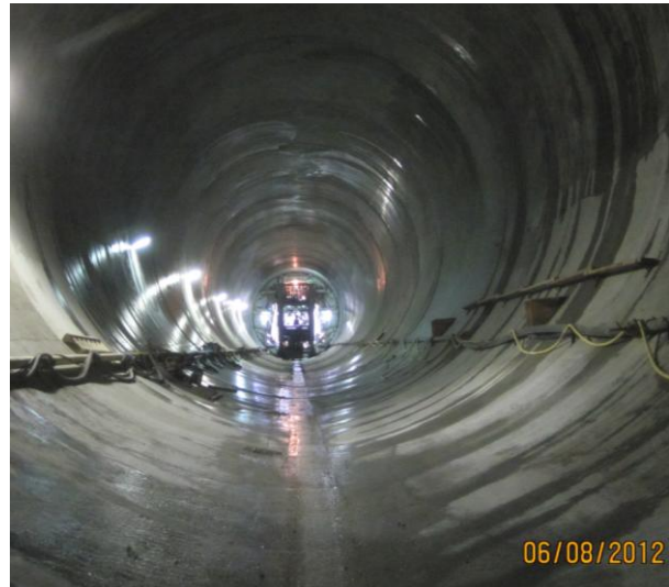
Figure 6. Finished concrete liner.
