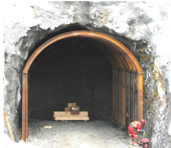
Figure 2. Portal and access adit development.
