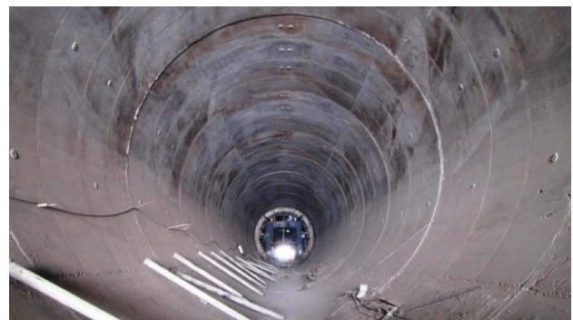
Figure 22. Internal view of concrete lining of tunnel
