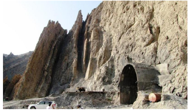
Figure 19. View of right diversion tunnel from Intake.
