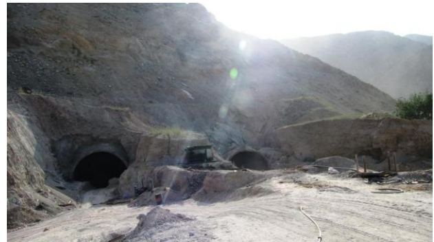
Figure 20. External views of diversion tunnels from outlet.
