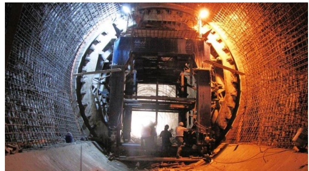
Figure 21. View of diversion tunnels construction.
