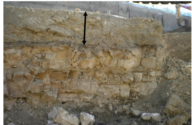
Figure 6: An excavation site in Calgary SW in which the weathered zone atop the bedrock is clearly visible.
