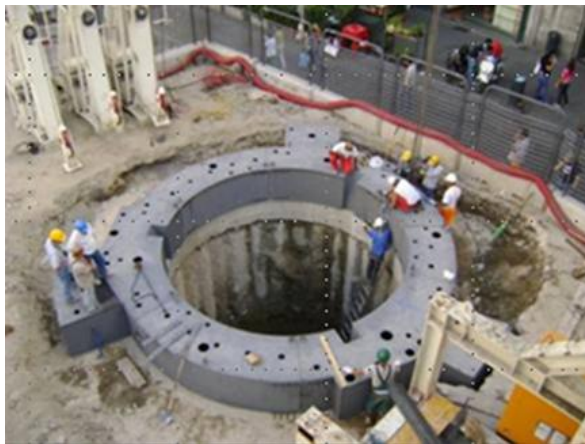
Figure 10. Reusable Ring Beam
