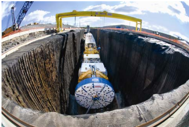
Figure 4. The 14.4 m diameter Main Beam TBM at the time of launch
