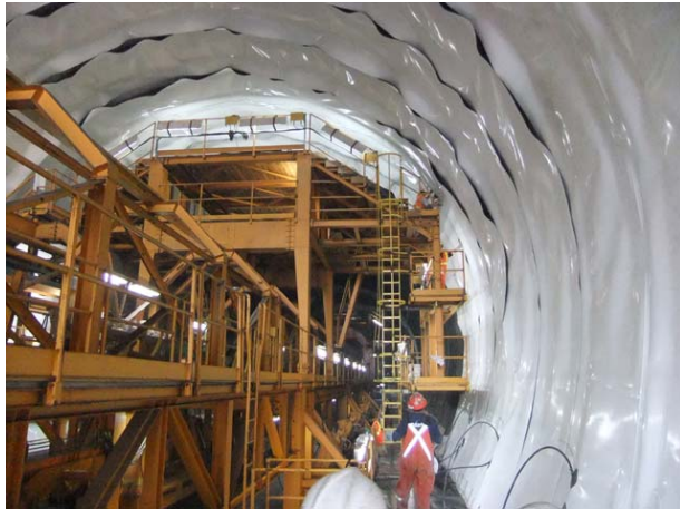
Figure 12. Waterproof Lining Installation
