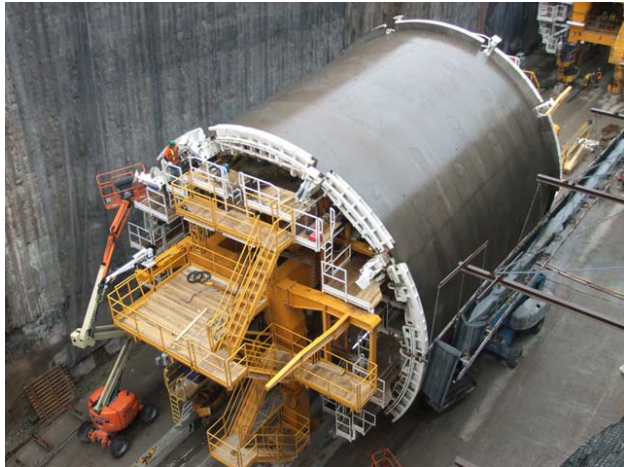
Figure 13. Concrete Lining Arch Form
