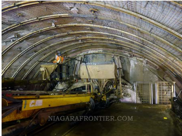
Figure 7. Revised ground support system
