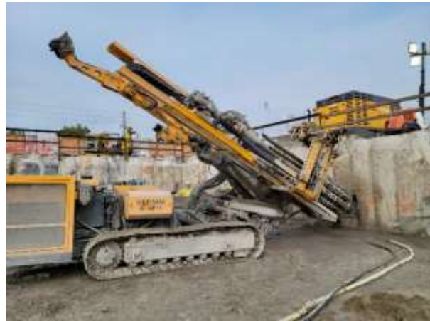
Figure 10: Tieback Drill Rig utilized at LS1 site
