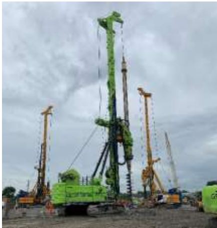
Figure 9: Secant Pile Drill Rigs at LS1 Site
