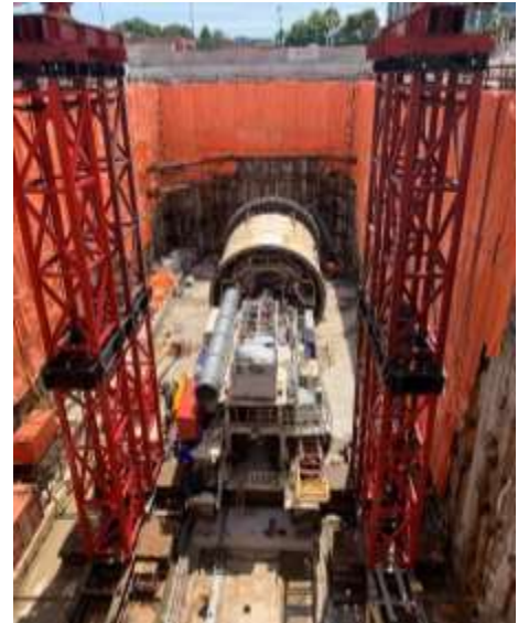
Figure 14: TBM and Gantry 1 in shaft
