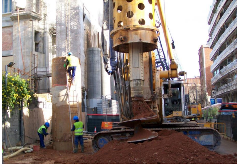
Figure 10. Pile Wall construction in front of Glory Façade
